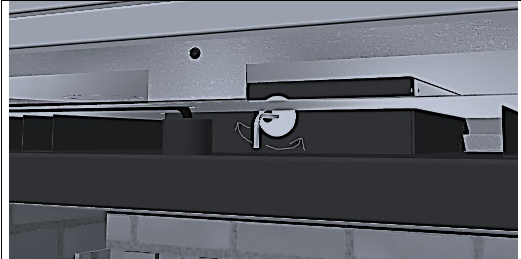
Figure 4-21 Exhaust Damper Adjustment
